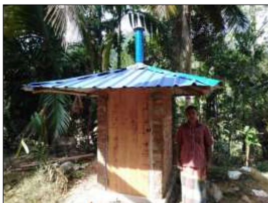
Fig. 3. Construction of a Rubber Processing Center – A K Konara (Gampaha range)
